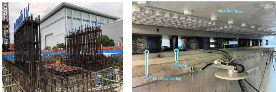
Fig 7 Pictures of PC Strand during construction and after completion
